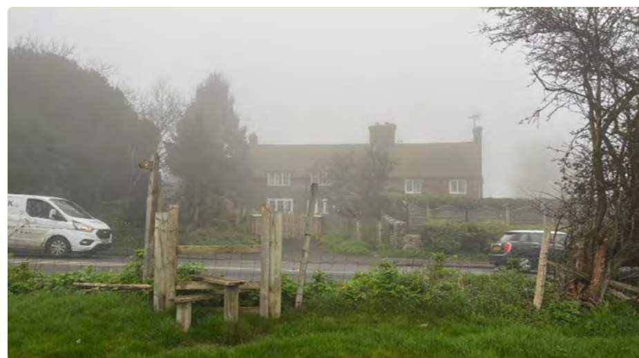
▲ Plate 8: View from the north-western extent of the site towards the asset's southern elevation, through the stile used for public footpath access into the site.
