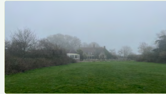
▲ Plate 1: Lower Barnhorne's south-western elevation facing over a site parcel proposed as a 'soft setting' to the Listed Building. On concept plan: pink circle indicates location of asset and red arrow indicates location of photo.
