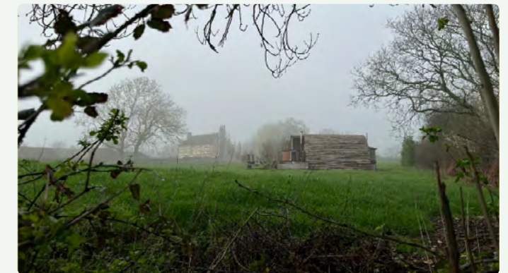
▲ Plate 4: The southern elevation of Upper Barnhorn Manor and glamping pods glimpsed through a gap in hedgerow vegetation along the northern site boundary. On concept plan: pink circle indicates location of asset and red arrow indicates location of photo.
