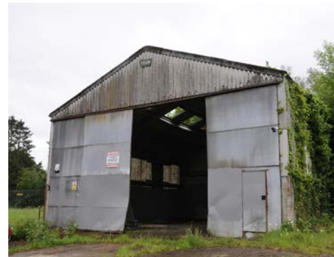
The Engine Shed, viewed from the south-east
