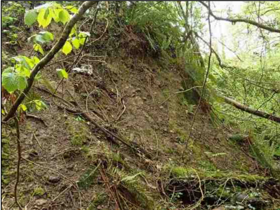
Plate 2. A substantial recent stream bank collapse in Coneyburrow Wood.
