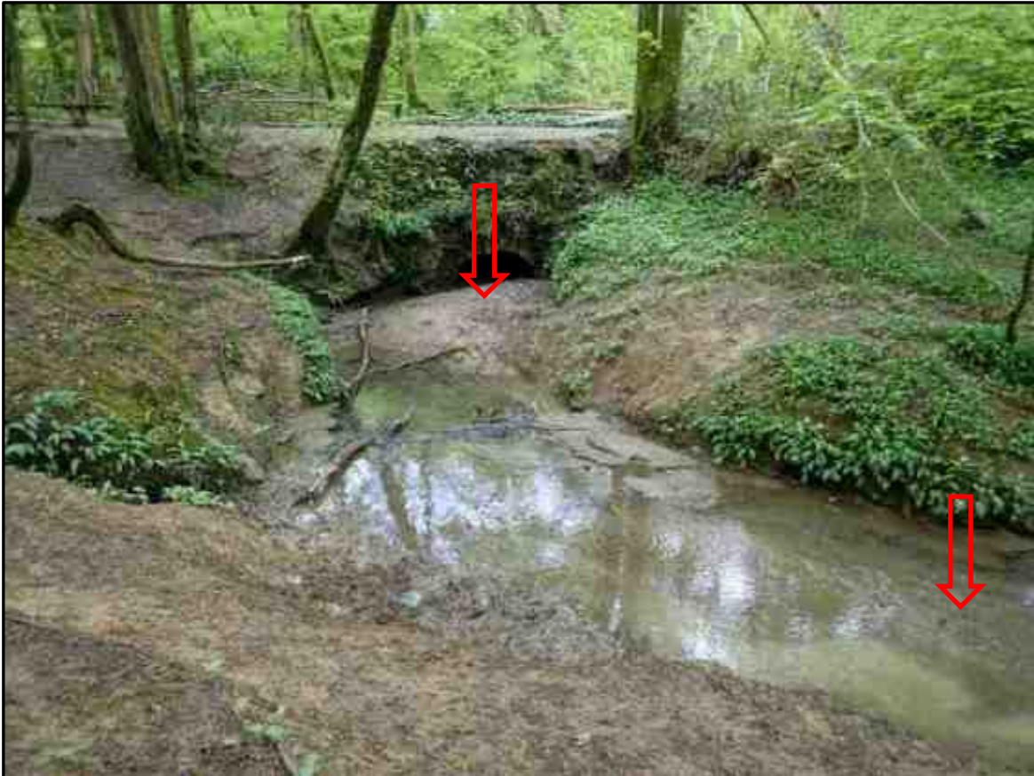
Plate 3. Banks severely eroded by dogs/people near the footbridge in Marline Wood. Prominent silt bars are also present above (arrowed) and below the bridge
