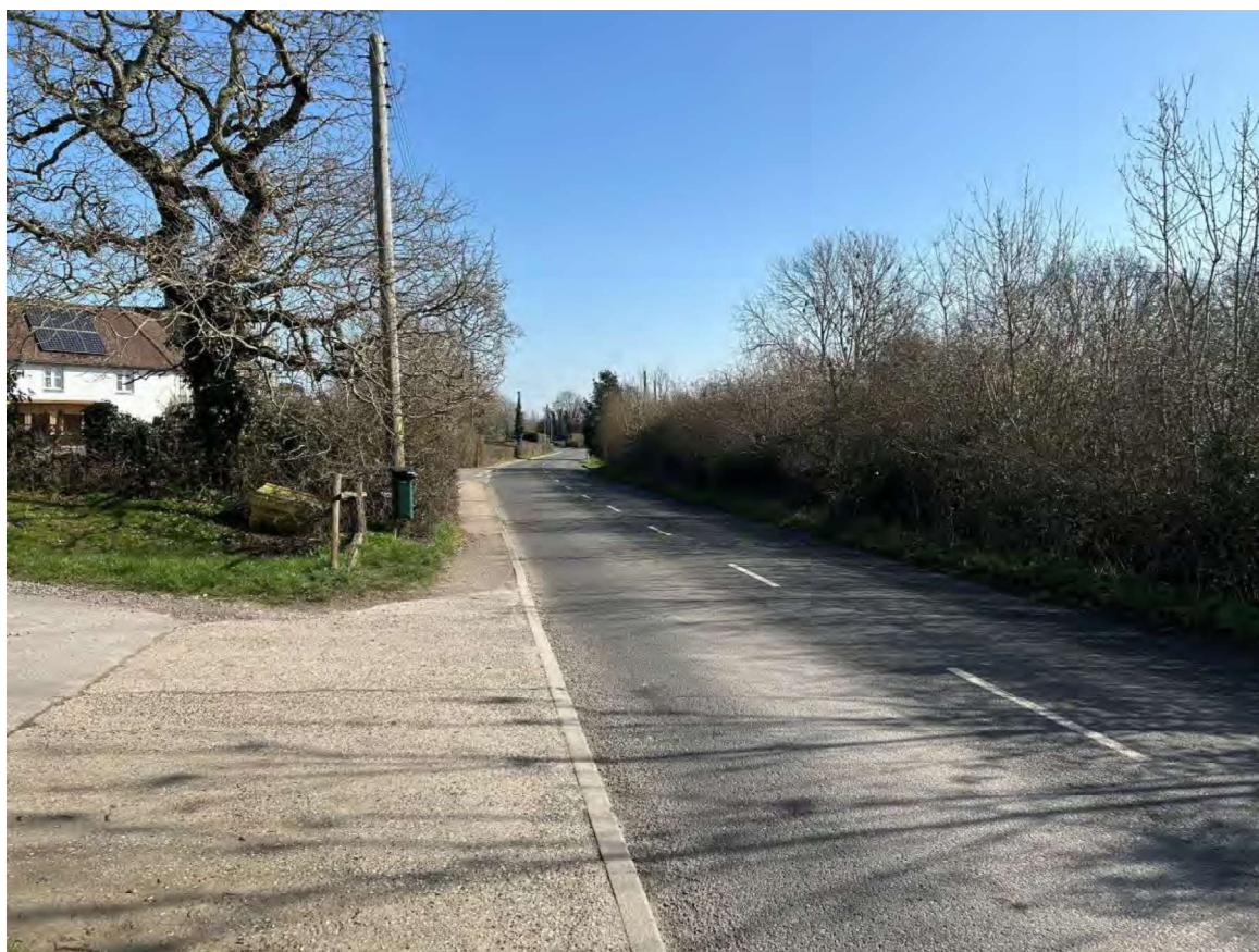
Existing Highway Conditions on Northiam Road
