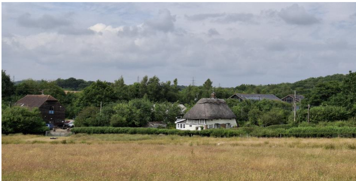
Figure 5: Wheel Cottage within its setting. The Business Park buildings are seen to the left and rear of the listed building. The subject site is located approx. 200m rear of the viewpoint and physically separated by 3 (unlisted) dwellinghouses and their residential curtilage.
