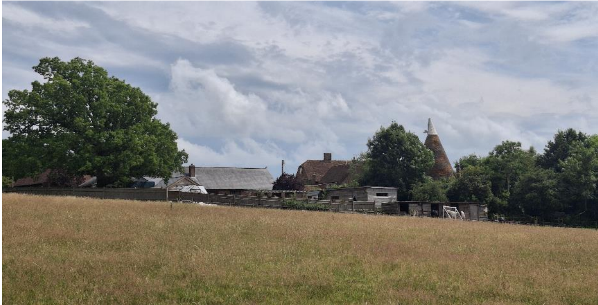
Figure 3: View of the Church Place Farmhouse from the subject site. Note the modern development (Parlour, Tennis court and outbuildings to the front). The roof of the Church Place Barn is seen to the left.
