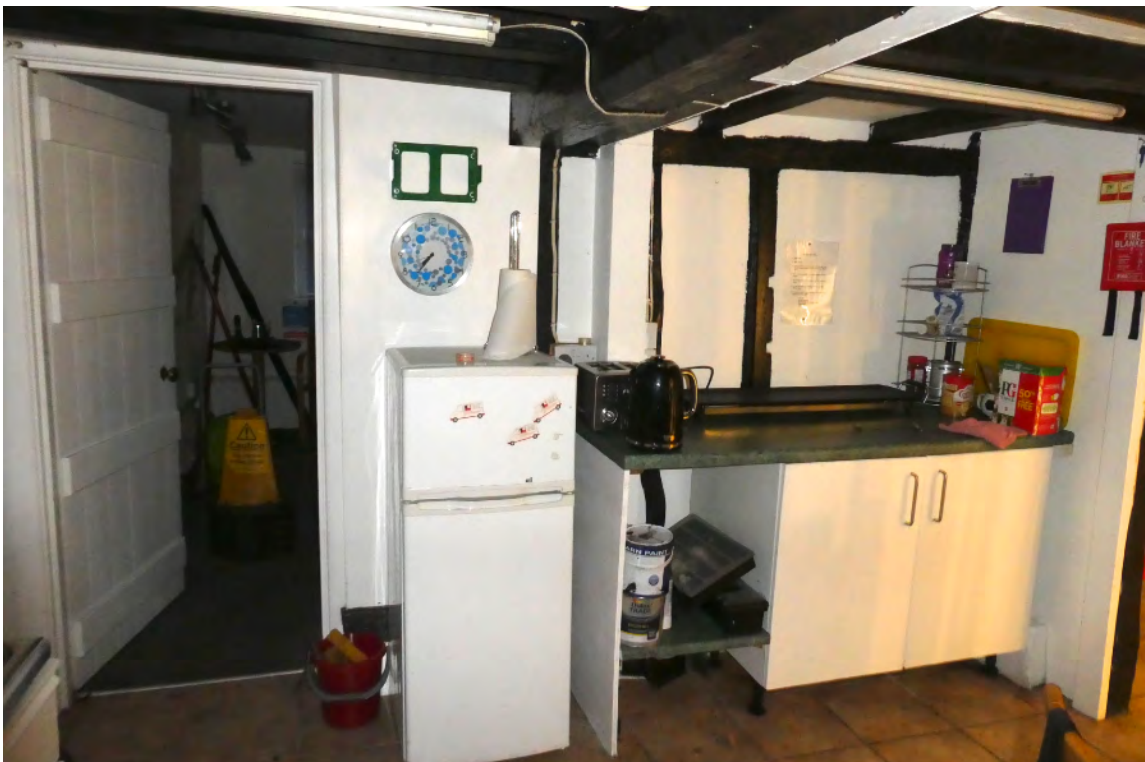
4. Internal door proposed to be blocked left.
