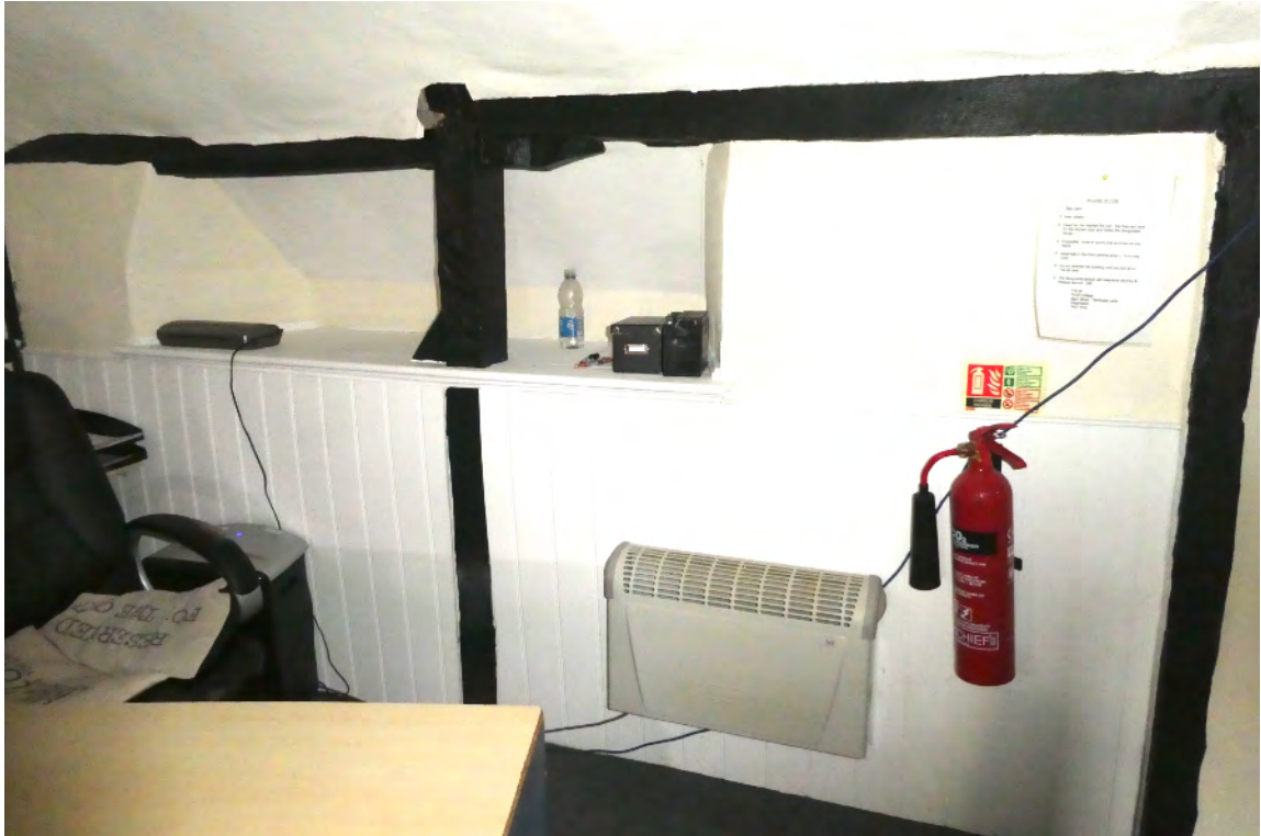
11. Inside rear wall of main frame at first floor showing phase 1 rear west post of main frame centre left with main eaves plate over. Phase 2 eaves plate lapped over right.
