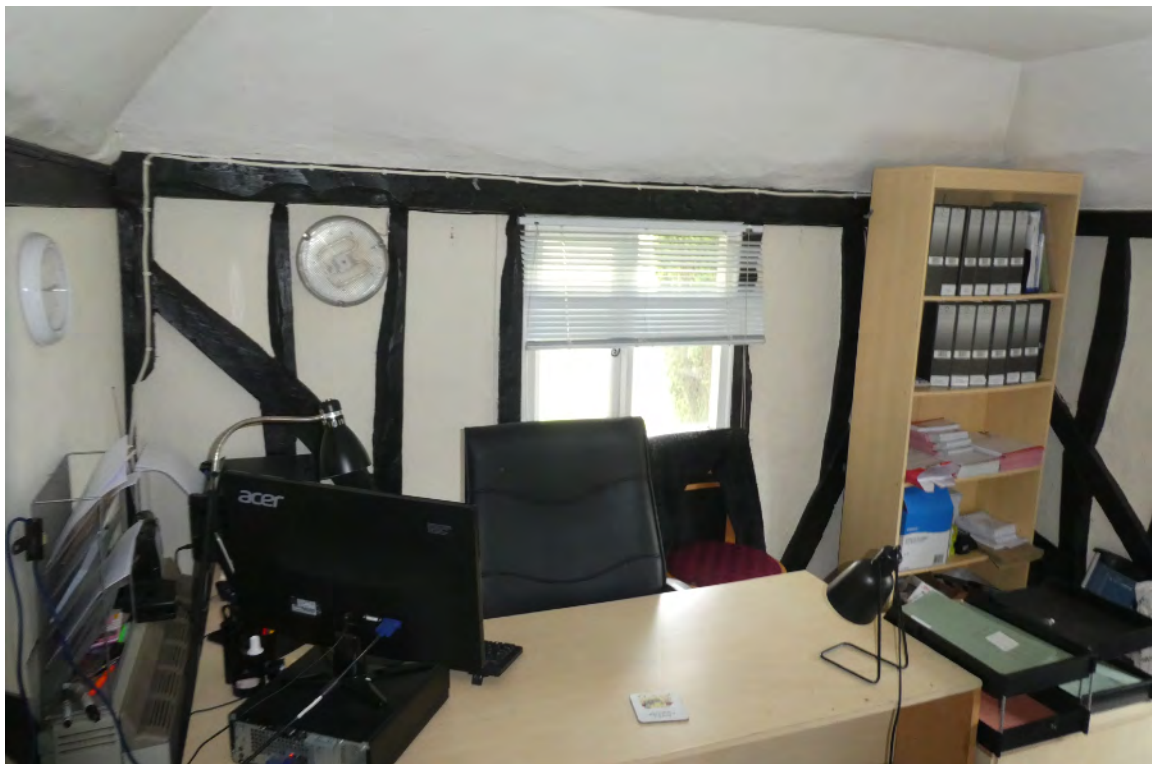
18. Phase 2 added west bay looking west in first floor chamber showing raking strut and stud construction and bowl shaped jowl to head of principal post left.
