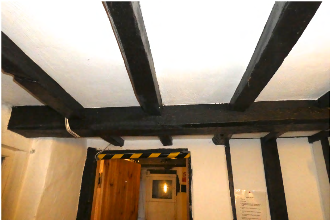
16. First floor cross beam and joists over phase 2 west bay.
