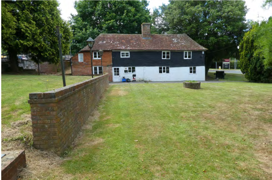
1. Front (north), phase 3 extension left.
