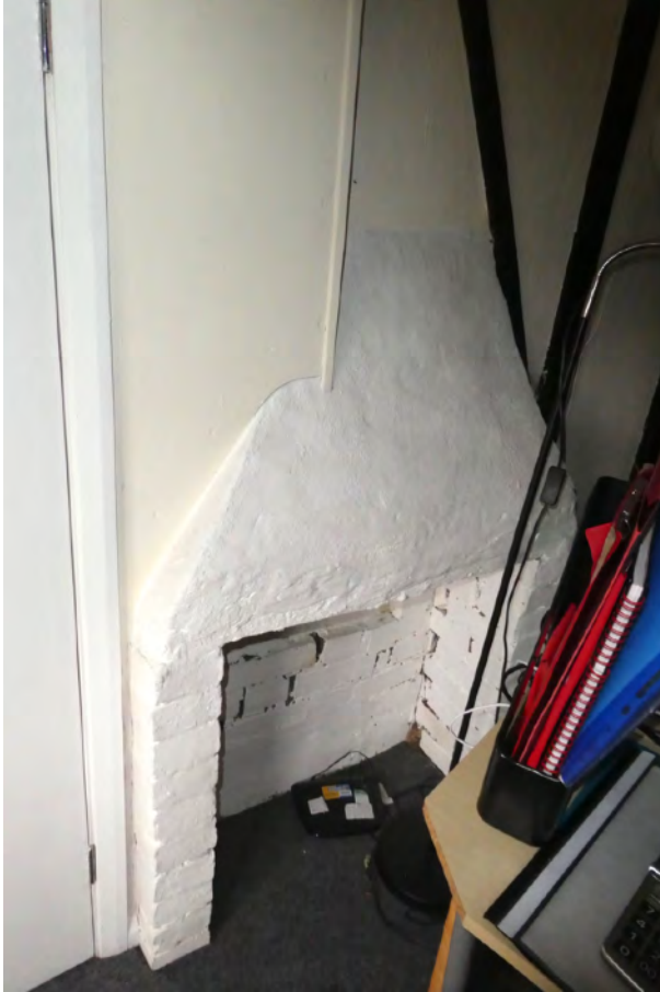
17. Phase 2 west cottage first floor fireplace.
