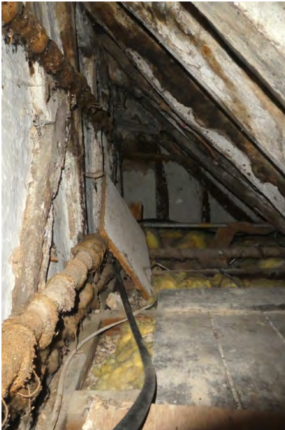
11. Inside rear wall of main frame at first floor showing phase 1 rear west post of main frame centre left with main eaves plate over. Phase 2 eaves plate lapped over right.
