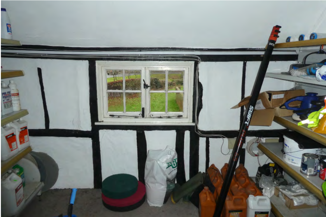
9. Inside front wall of phase 1 services first floor chamber showing slender small square panel framing with interrupted midrails with raised cill for window in original position.
