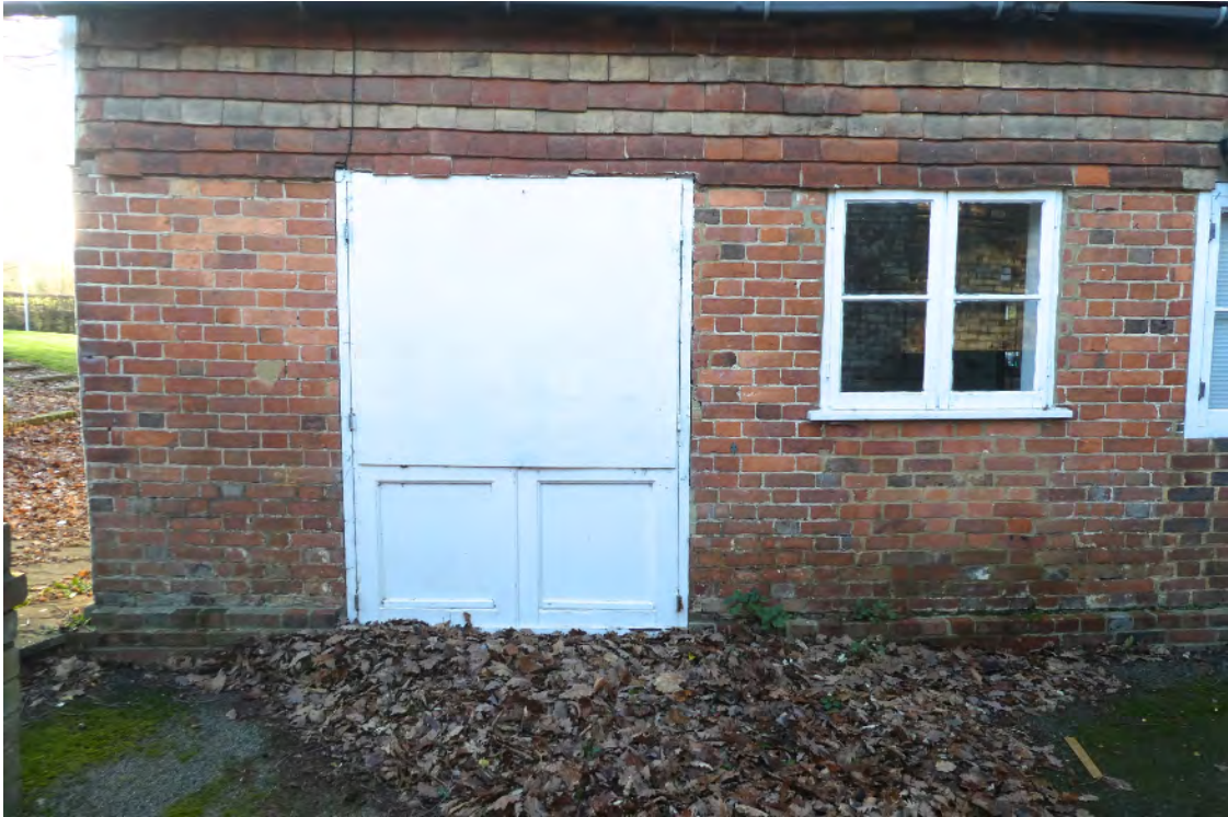
3. Former cafe entrance doors at east end proposed to be reinstated as French doors.
