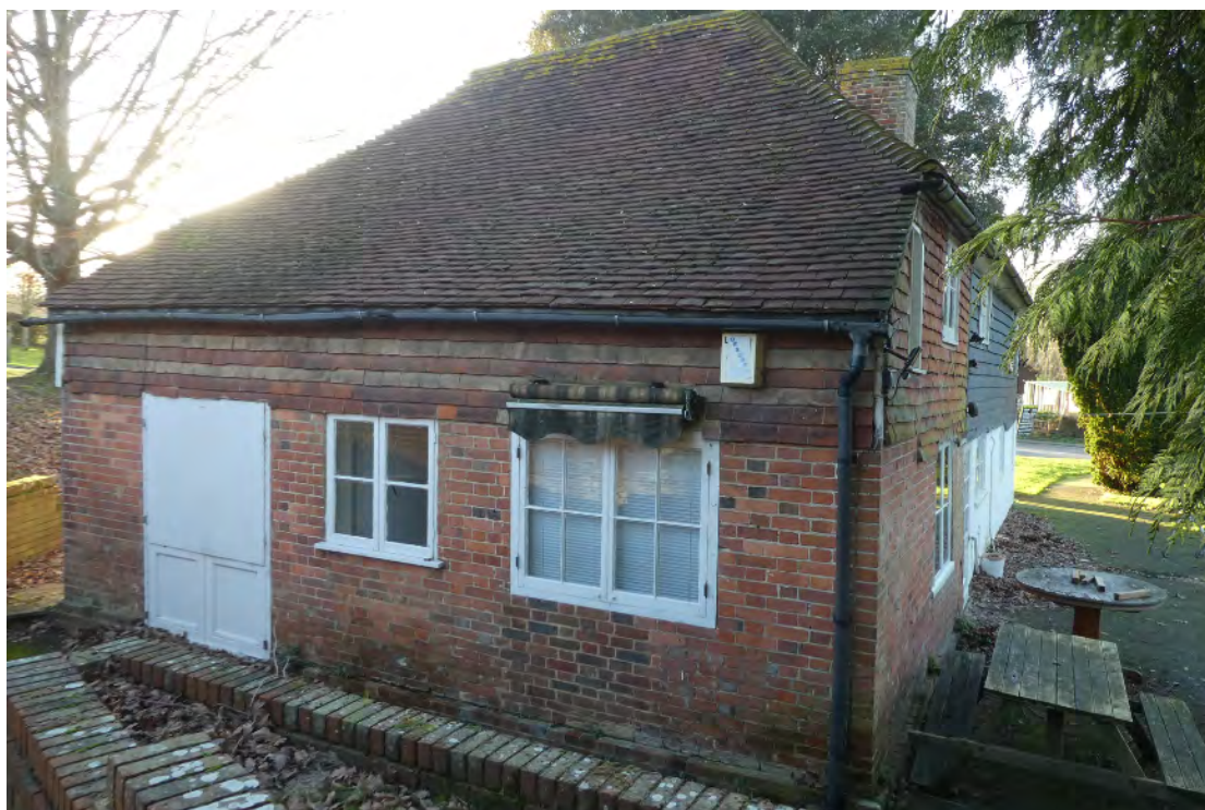
2. Side (east) showing phase 3 extension.
