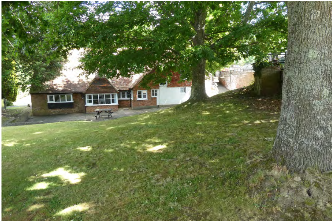
9. From south from edge of supermarket drive to be screened by hedge planting, oak trees right to remain.
