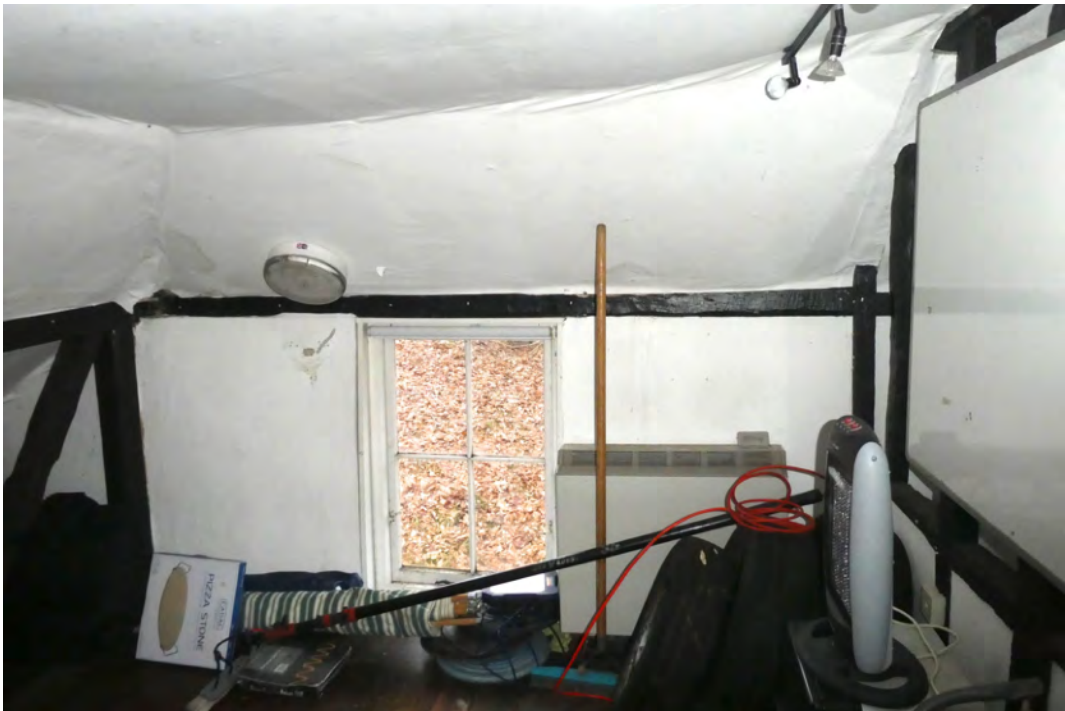
20. Phase 3 rear first floor room looking to rear.
