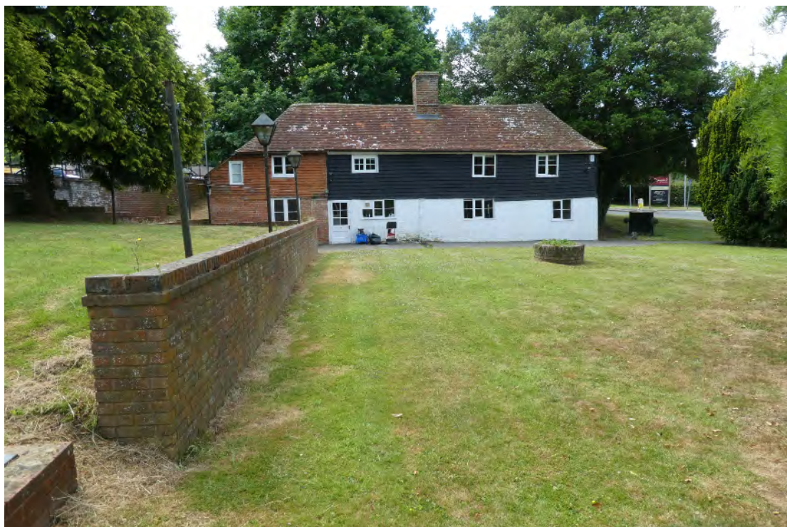
1. Front (north), phase 3 extension left.
