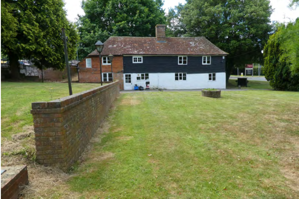
7. Pond Cottage from the north, site of proposed retirement flats left beyond retaining wall. Cottage to right of wall to remain visible from the main road.
