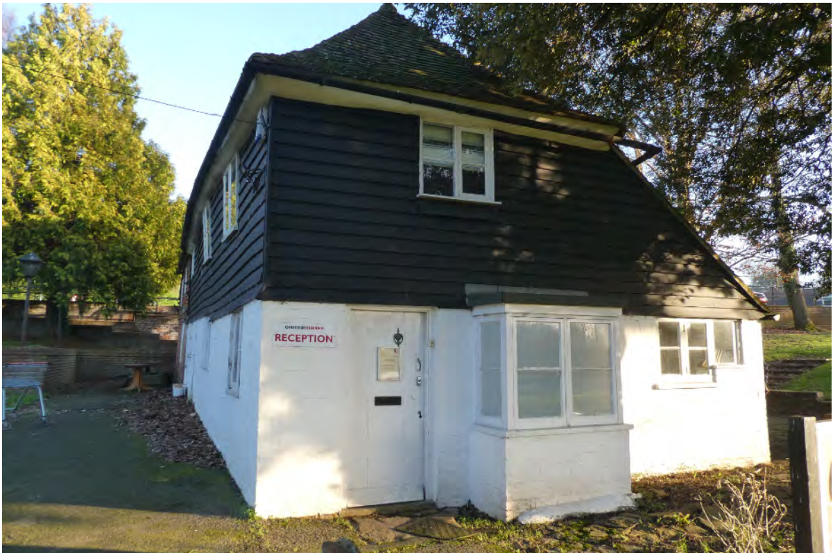
4. Side (west) showing phase 2 west extension.
