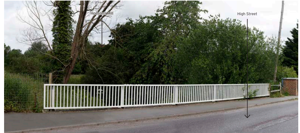
Viewpoint 1: View west towards the Site from High Street
