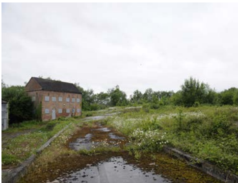
View west towards the Oast House from within the Site
