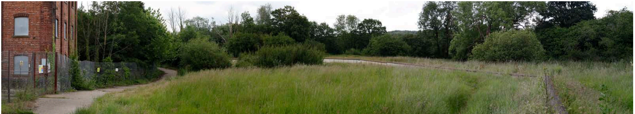
View across grassland to the south of Hodson's Mill with flood defences visible
