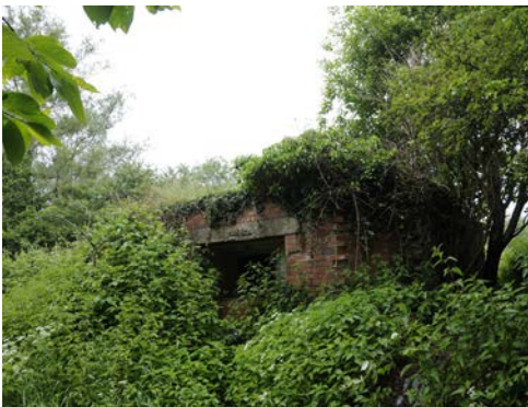
Pillbox as seen from the south-east
