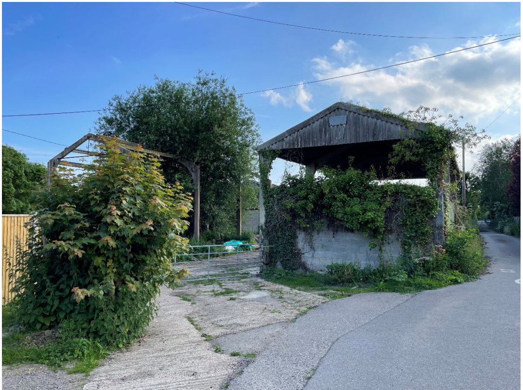
Plate 8 Looking south to the modern barns
