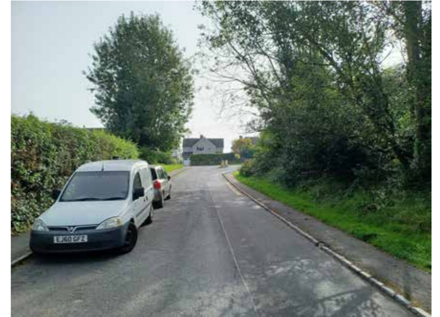
Photo 14: View East from Virgins Lane
